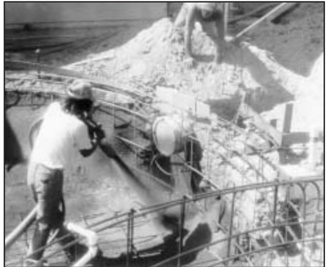
Fig. 8 BADUJET Ready for Guniting
